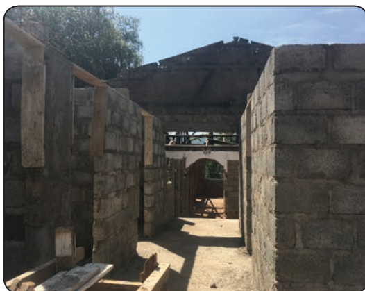
Repairs and renovations underway at the Bomet Annex – March 2017
