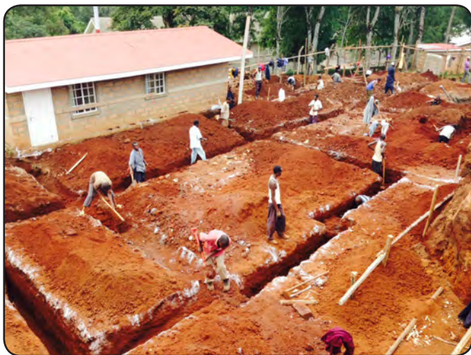
Foundation underway for housing project
